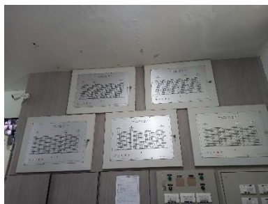
Graphic Annunciator Fire Alarm System
